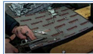
**Step 5: Apply the selected material to the surface.** Remove the pre-applied protective layer from the adhesive coating of the material and apply it to the target surface. Thoroughly press down from the center to the edges of the section.
